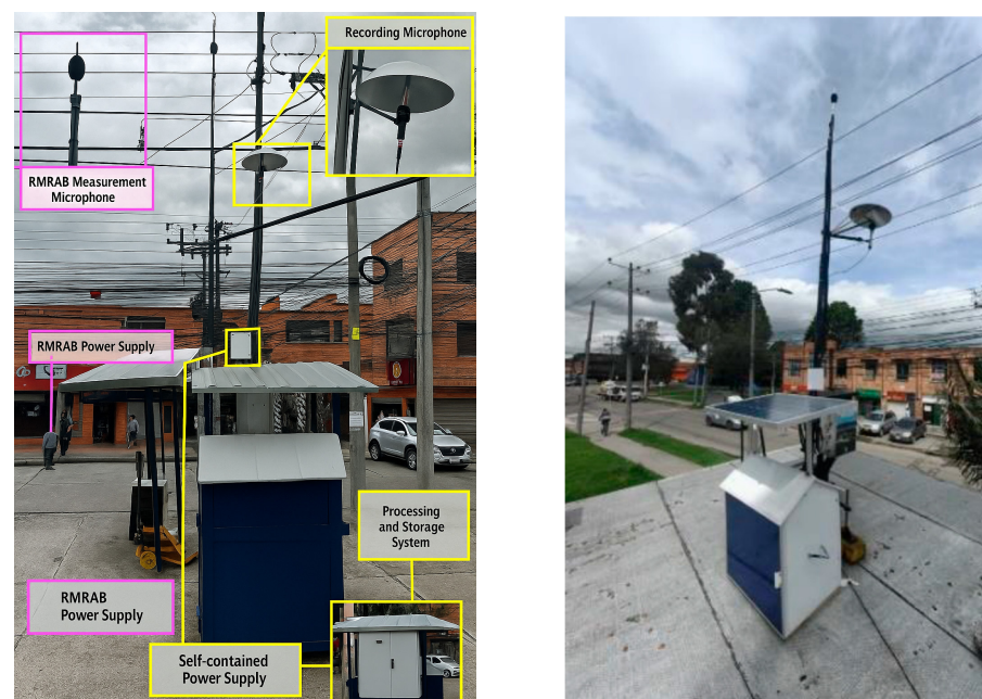
Figure 8. Monitoring station installation.
